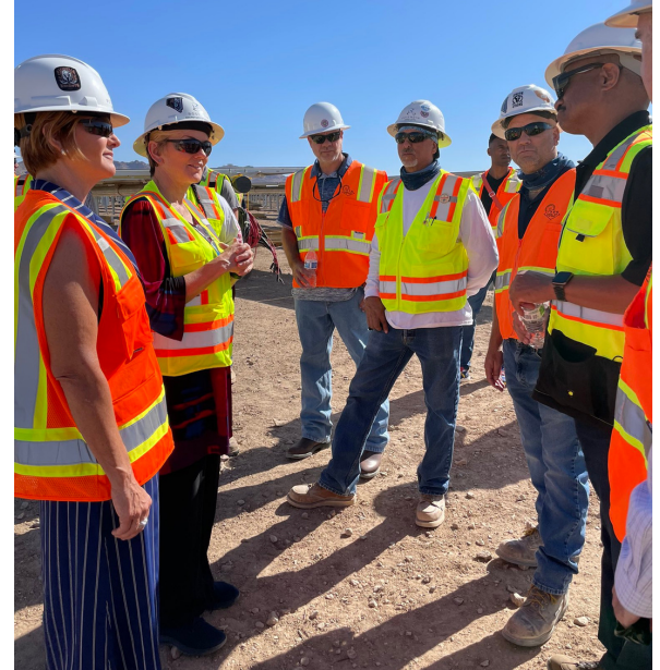
Energy secretary Jennifer Granholm toured the solar project under construction with the assistance of Las Vegas Local 357 members.
