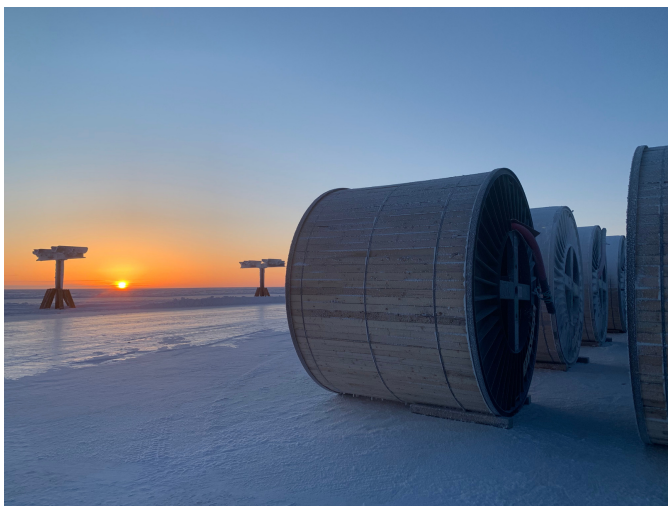
Alaska's Willow oil and gas project is providing jobs to dozens of Anchorage Local 1547 members.
